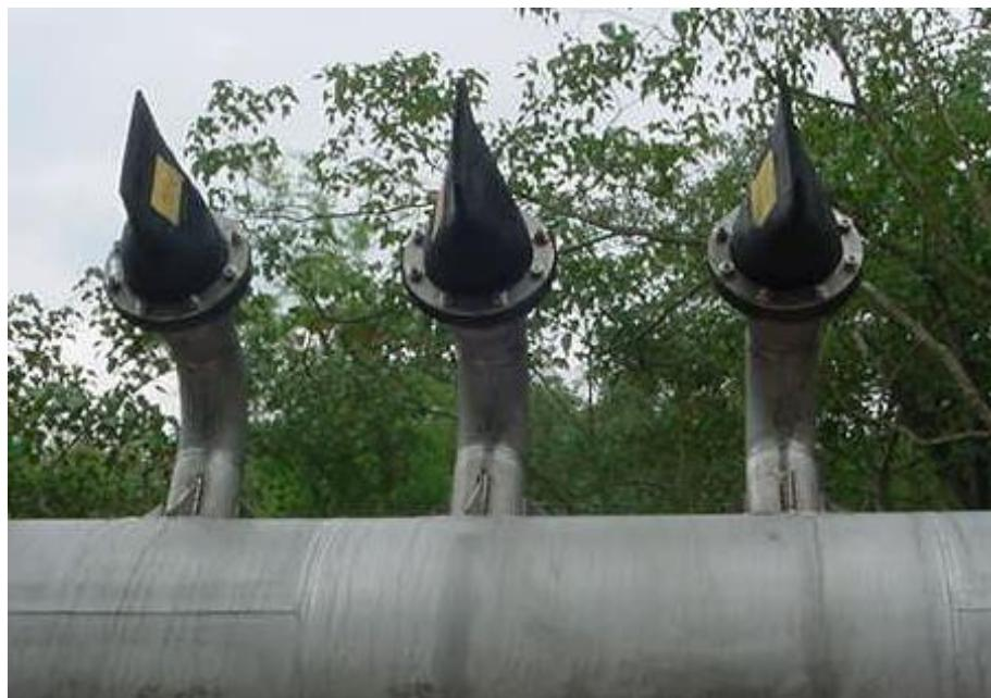
**Figure 4 – Exemple of special check valve (duckbill type).**
