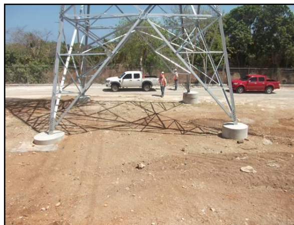
Photo 4-3. Typology of pedestals on the foundation where the metal structures of the towers will be anchored.
