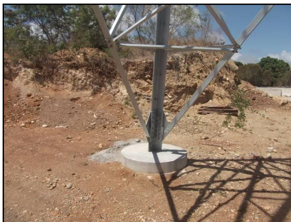
Photo 4-3. Typology of pedestals on the foundation where the metal structures of the towers will be anchored.
