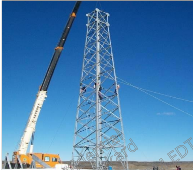
Photo 4-4. Steel tower hoisted with crane.
